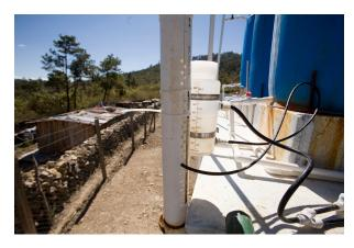
Alum and chlorine are dosed using a flow controller (FC) developed by AguaClara. The FC is a small jar fitted with a plastic float valve on the inlet, and a calculated length of tubing on the outlet. The float valve ensures a nearly constant head, while the elevation of the discharge of the exit tubing determines the total head loss, and hence flow rate.
