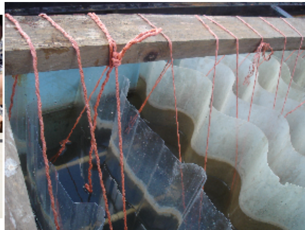
beam and string system to lift all flocculator baffles simultaneously closeup
