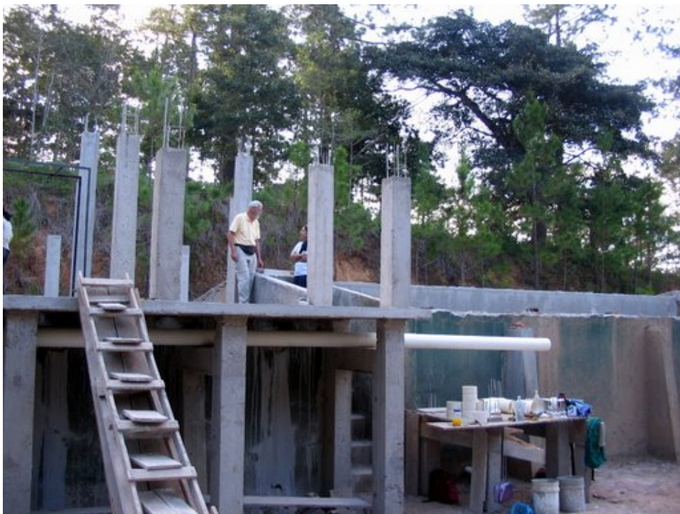
Photo of the Marcala sedimentation tank under construction.
