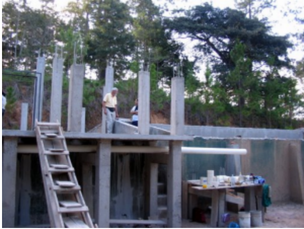
Marcala Plant (sed/flocc on left, distribution tank on right)
