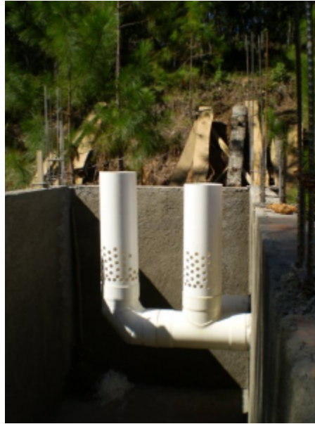
Flow control from grit chamber into flocc tank
