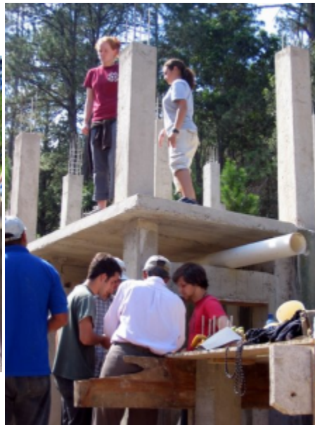
Laying pipe from sed tanks to leveling tank
