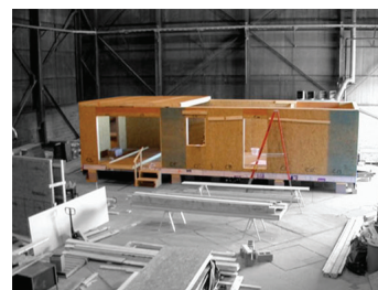
The 2005 house being built
