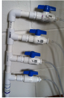
Figure 4: PVC Manifold
