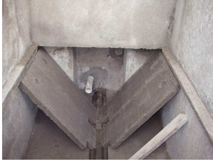
Figure 6: Photo of Inlet Slopes Construction
