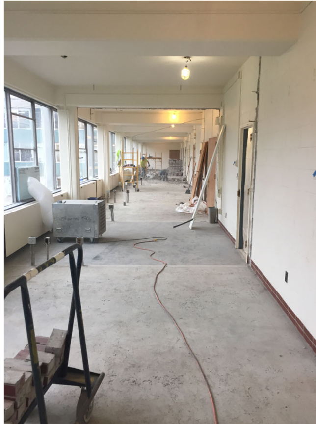
3 rd floor offices with walls demoed
