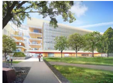
New Building Replaces Hollister North Wing
