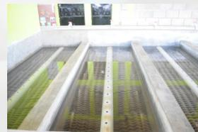
1. Water entering the plant is dosed with a chemical coagulant that will adhere to suspended particles.
