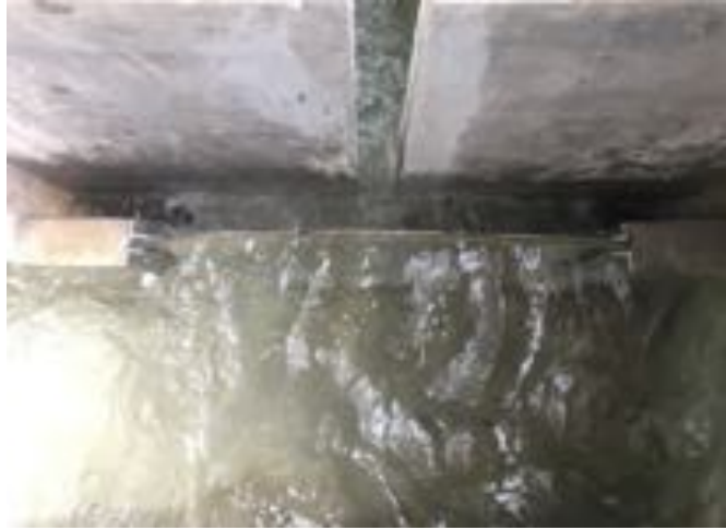
Figure 6: Las Vegas weir system is warping from water pressure
