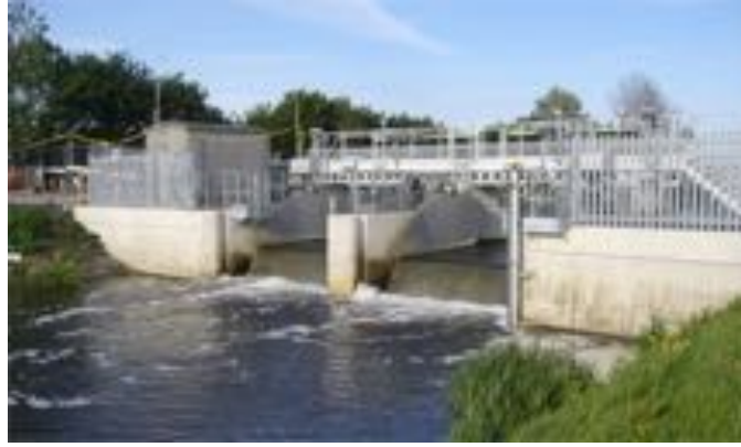
Figure 3: Parallel Weir System
