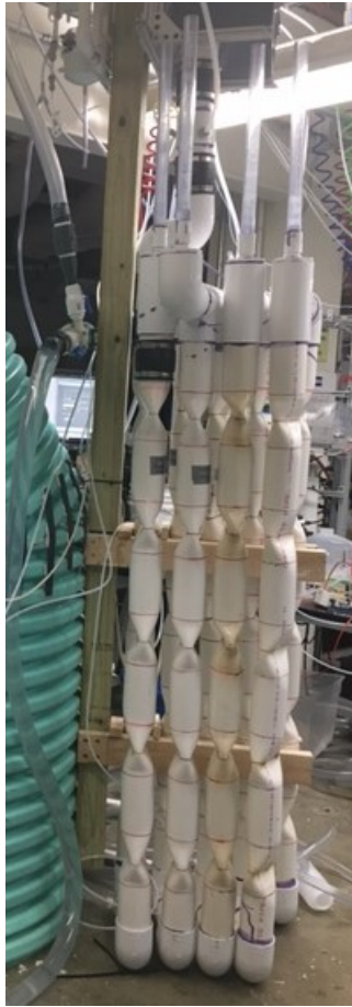
Figure 9: Flocculator of the 1 L/s plant.
