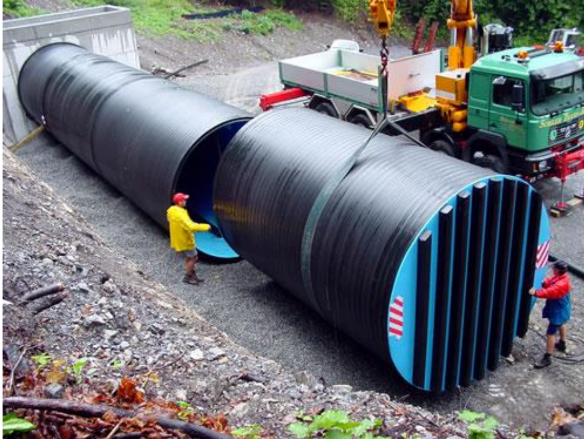
Spring box Switzerland (Polyethylene)
