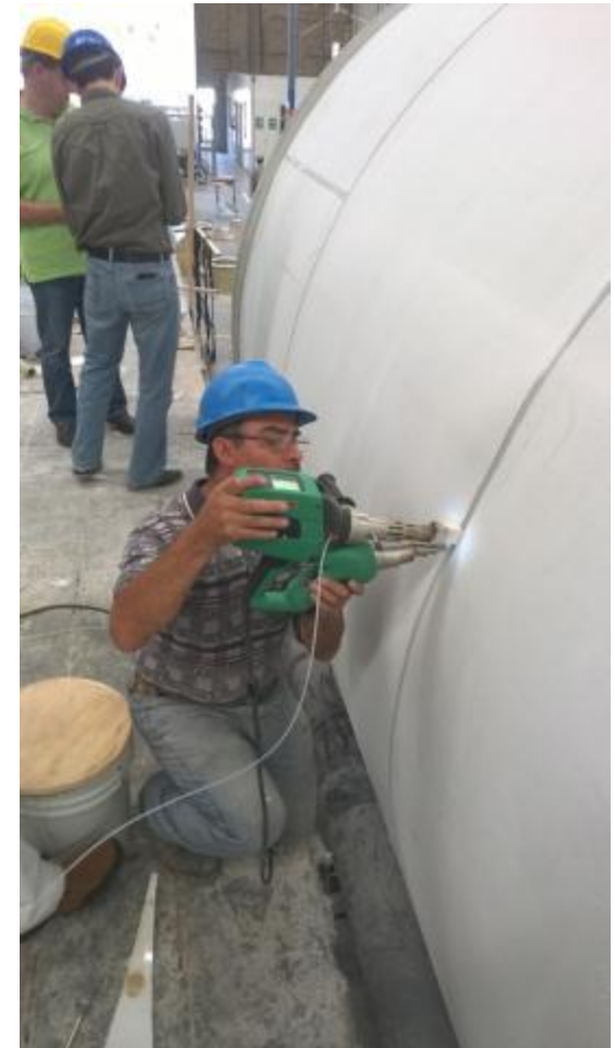
Water tank (Polypropylene) Fiberglas Konstruktion PP liner Mexico
