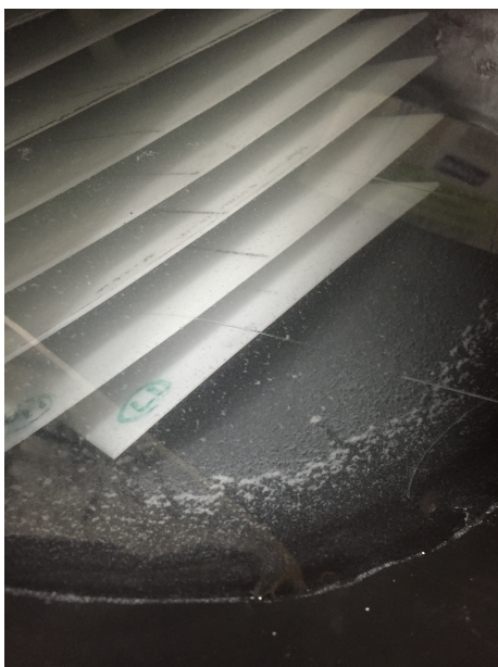
Figure 18: Once flocs are large enough to settle, they slide down the sloped walls of the tank down to the floc blanket.
