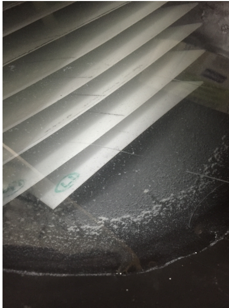
Figure 17: Once flocs are large enough to settle, they slide down the sloped walls of the tank down to the floc blanket.
