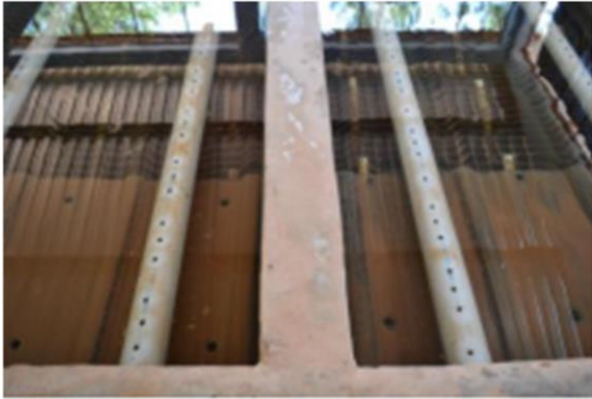
Traditional plant exit launder
