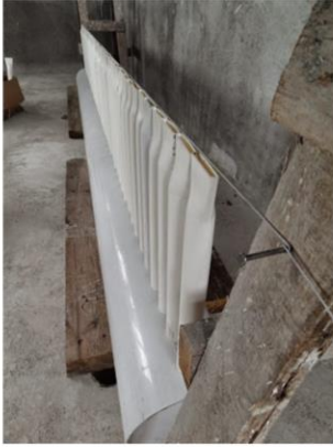
Full scale influent pipe in a traditional plant
