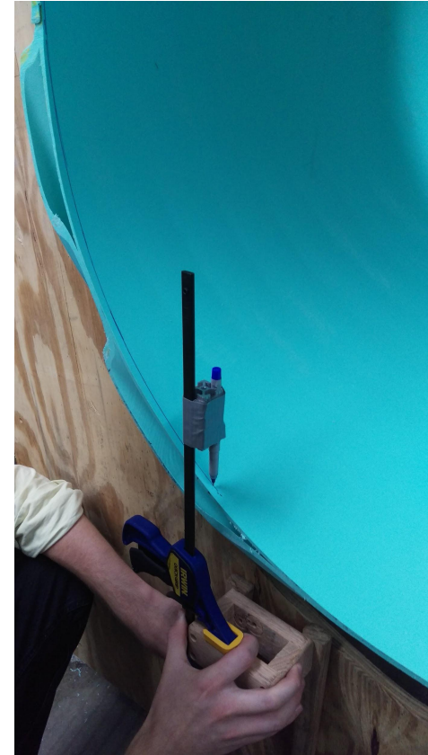
Using the jig
