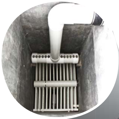
Rapid Sand Filtration with stacked geometry
