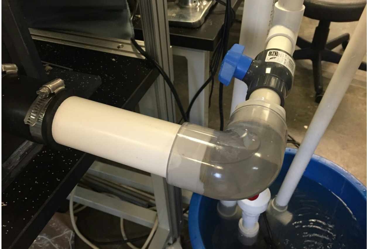
Figure 3: The bottom inlet modified by adding a valve.
