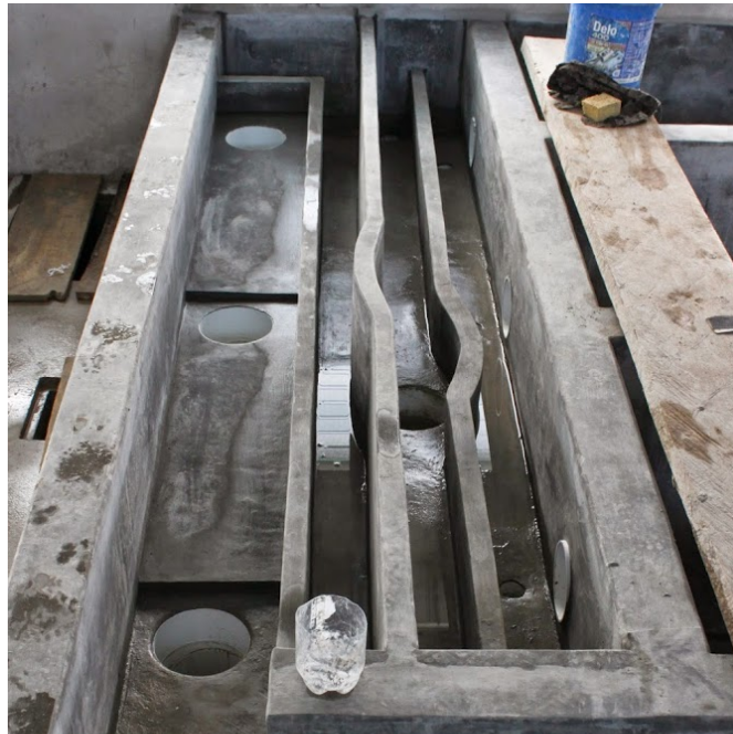
Figure 16: Exit Channel in Morocelí
