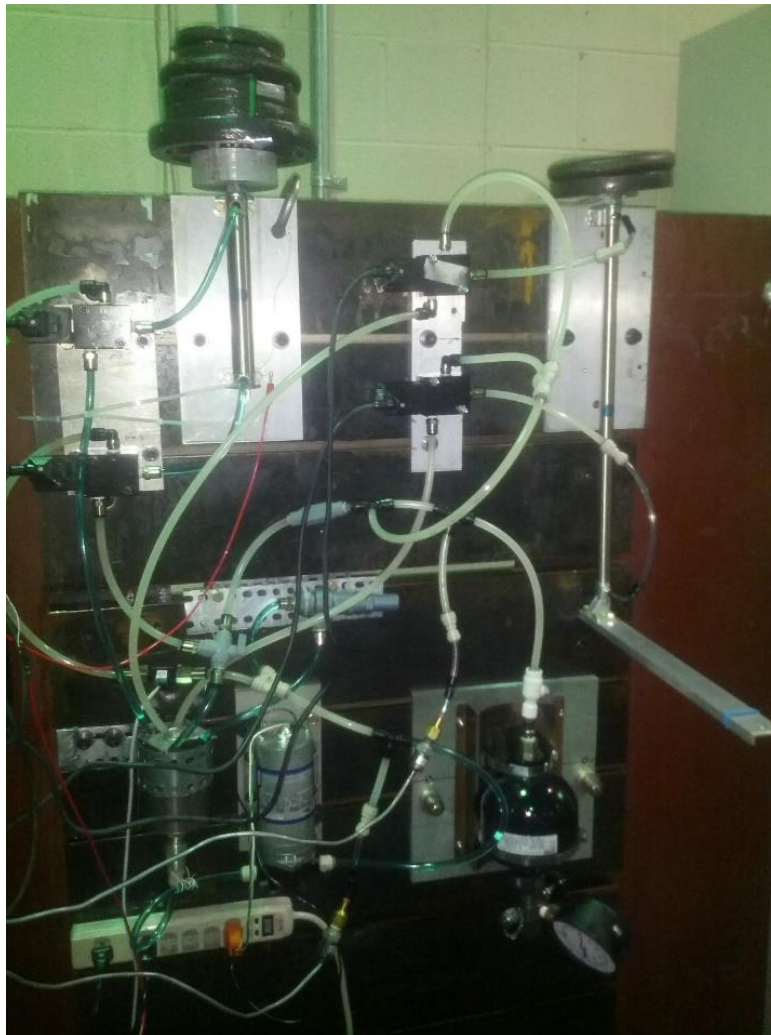
Figure 7: Photo of dangle and regenerative braking test circuit.
