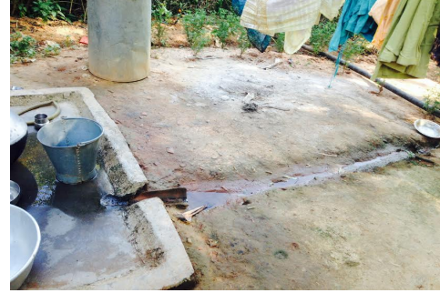
Fig 10. (Left) In the current platform design in place, water flows directly from the platform to surrounding agriculture. Fig 11. (Right) In other platform designs, a divot in surrounding soil allows water to flow from the platform to slightly more distant agriculture.
