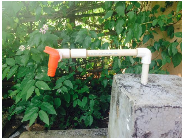
Figure 22: Pipe from distribution system and tap, including two 90 degree elbows.
