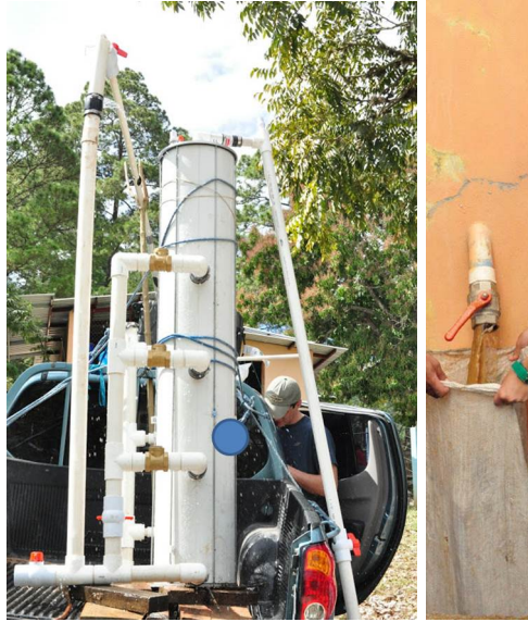
Figure 4: Sand drain for full scale SRSF (right) and proposed sand drain location for LFSRSF (left).
