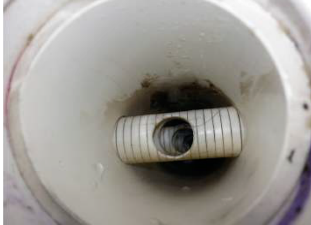
Figure 10: A view down the trunk (with slotted pipe) that shows the hole machined so water can flow into the branch pipe from the trunk line
