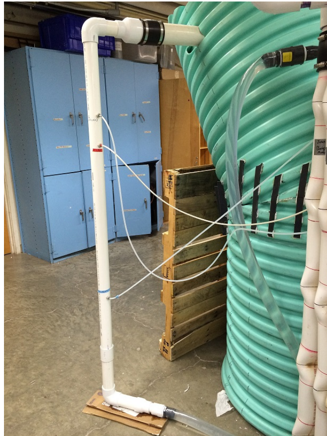
Figure 5: Sedimentation Outlet of 1 L/s Plant
