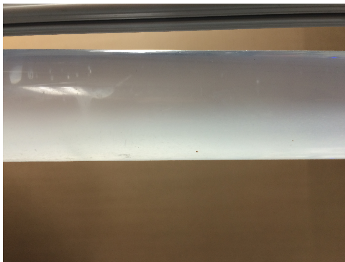
Figure 11: Clay Settling in Flocculator Effluent Tube
