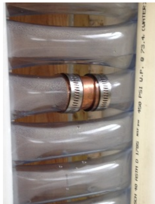
Figure 1: Flexible Tubing Connectors
