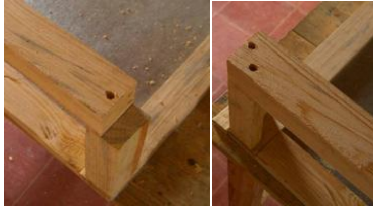
Figure 2: Left- One 3" screw is used to attach the side of the frame to the front column. Right- Two 3" screws are used to attach the side of the frame to the rear column
