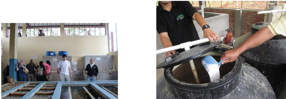
Figure 1: Coagulant stock tanks (blue drums in middle of the photo on the left) provide more than 24 hours supply of liquid coagulant. The chlorine tanks (photo on the right) contain a concentrated bleach solution made from calcium hypochlorite. The pipe mixing device used to stir the chlorine solution is visible on the right.
