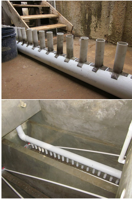
Figure 1: Spring 2011 version of the sedimentation tank inlet manifold and diffusers. These diffusers do not provide the continuous line source that is required to suspend all flocs that slide down the slopes of the sedimentation tank. In addition, the flat sludge drain cover does not provide the geometry for a jet reverser that can easily suspend the settled flocs.
