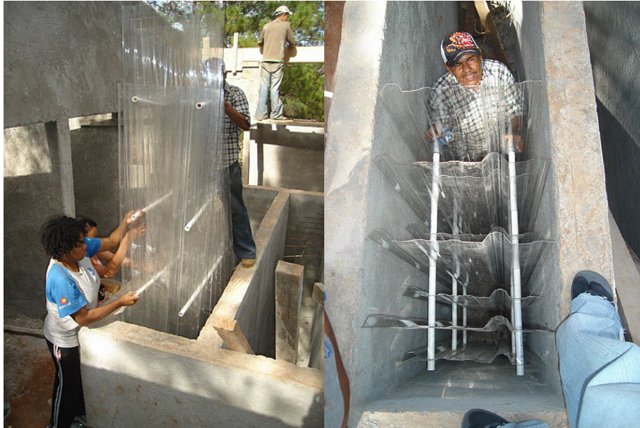
Figure 1: Floc baffle construction using corrugated plastic sheets and PVC pipes.
