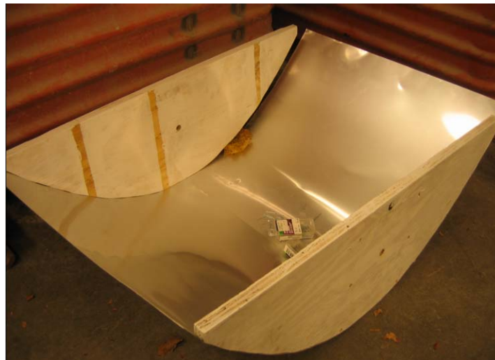
FIGURE 9. PARTIALLY COMPLETED PARABOLIC TROUGH COOKER.
