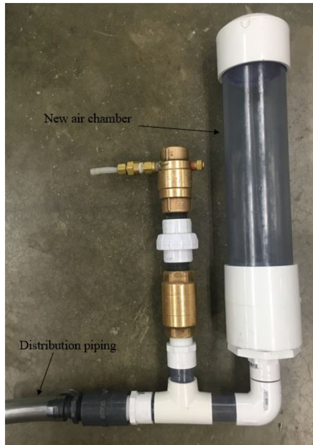
Figure 26: A second air chamber was installed next to the ram pump exit and behind the distribution piping in order to eliminate the vacuum effect.
