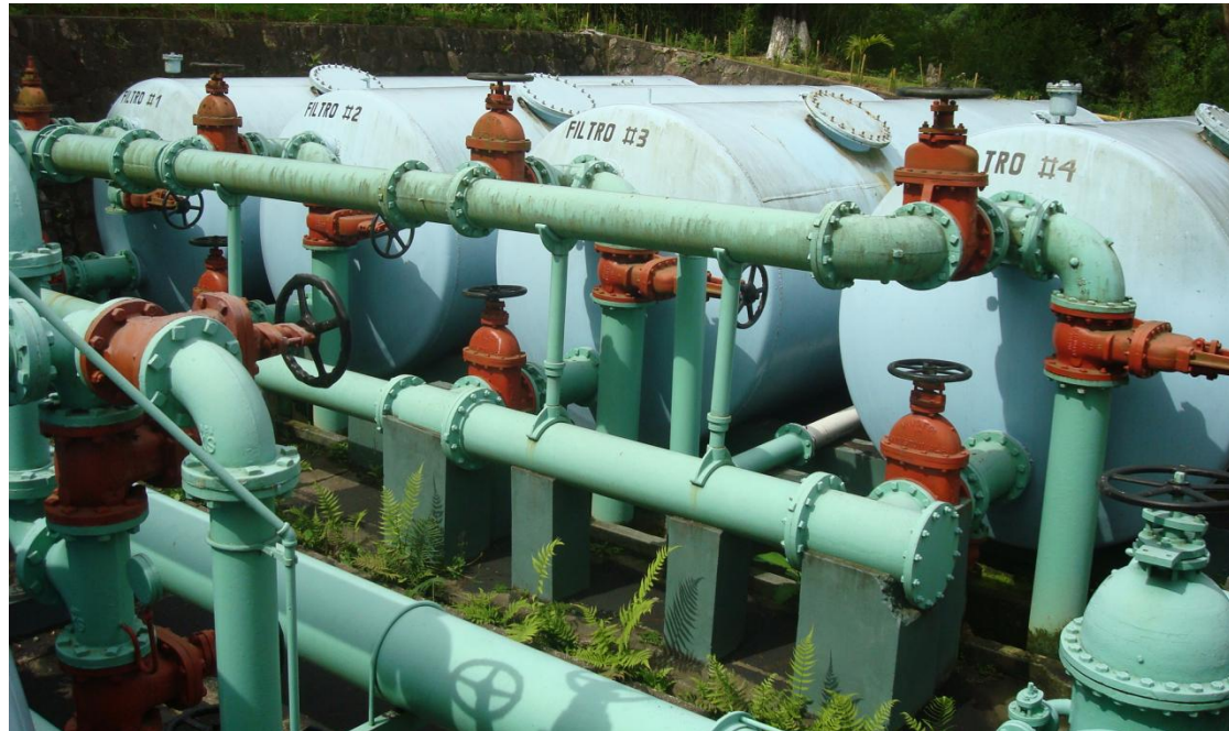
Abandoned rapid sand filters in Guatemala City
