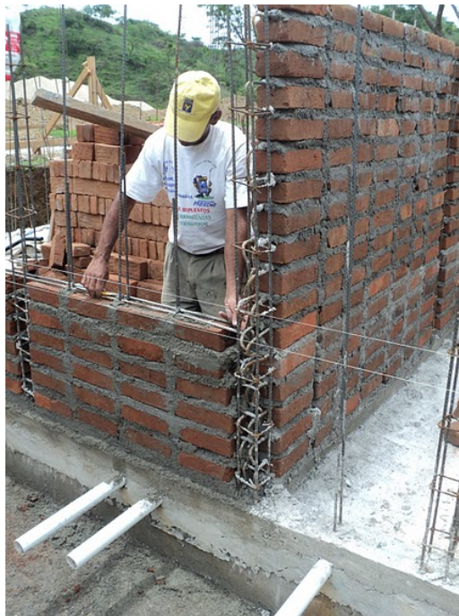
Figure 4: Wall and Column Rebar Configuration at the Alauca Water Treatment Plant
