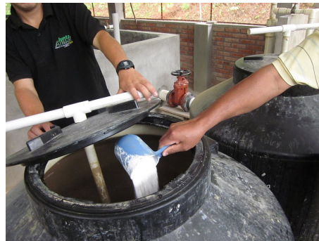
Figure 1: Coagulant stock tanks (blue drums in middle of the photo on the left) provide more than 24 hours supply of liquid coagulant. The chlorine tanks (photo on the right) contain a concentrated bleach solution made from calcium hypochlorite. The pipe mixing device used to stir the chlorine solution is visible on the right.
