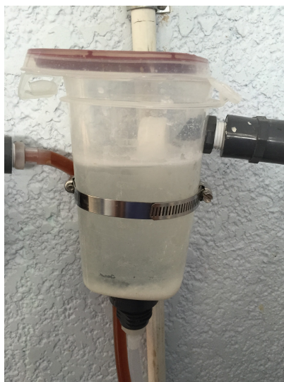
Figure 2: Current CHT design implemented in San Nicolás, Honduras. This CHT Design uses locally available plastic Tupperware as the tank with a custom float valve. There is evidence of chlorine stratification
