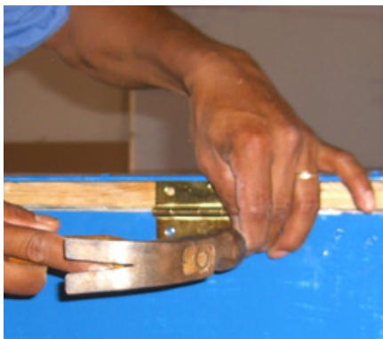
a. Use a nail to puncture the sheet metal before screwing in.
