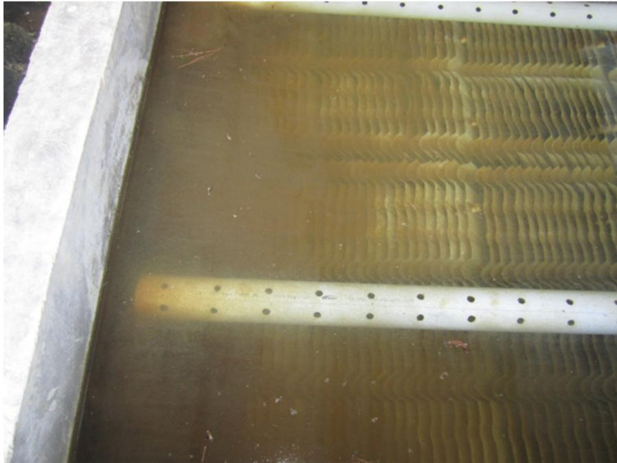
Figure 10: Visible flocs above Marcala's Tank 4's plate settlers
