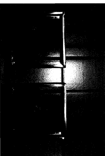
Fig. 17.3. A set of emergency shutoff valves for oxygen and nitrous oxide in a central pipeline system for medical gases in a veterinary teaching hospital. These valves should be placed strategically throughout the gas distribution system to control the flow of gases during emergencies or maintenance.
