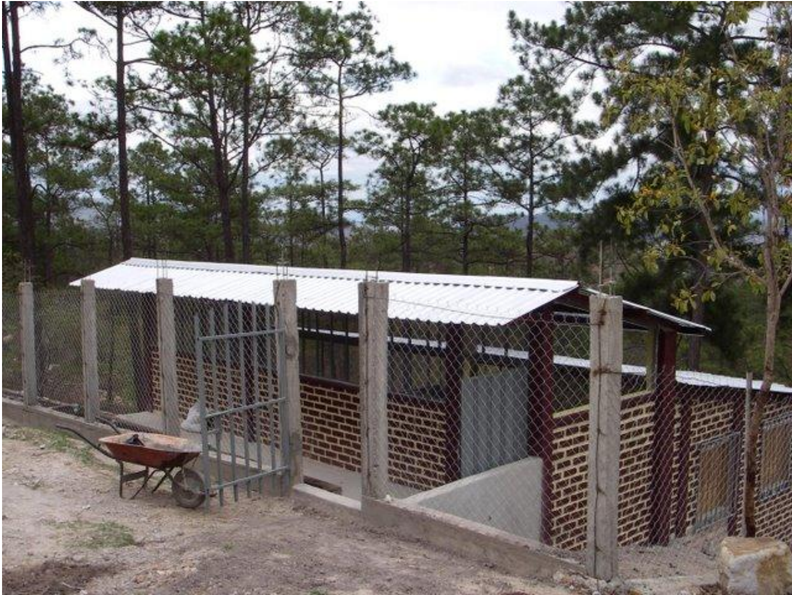
Constructed AguaClara water treatment plant
