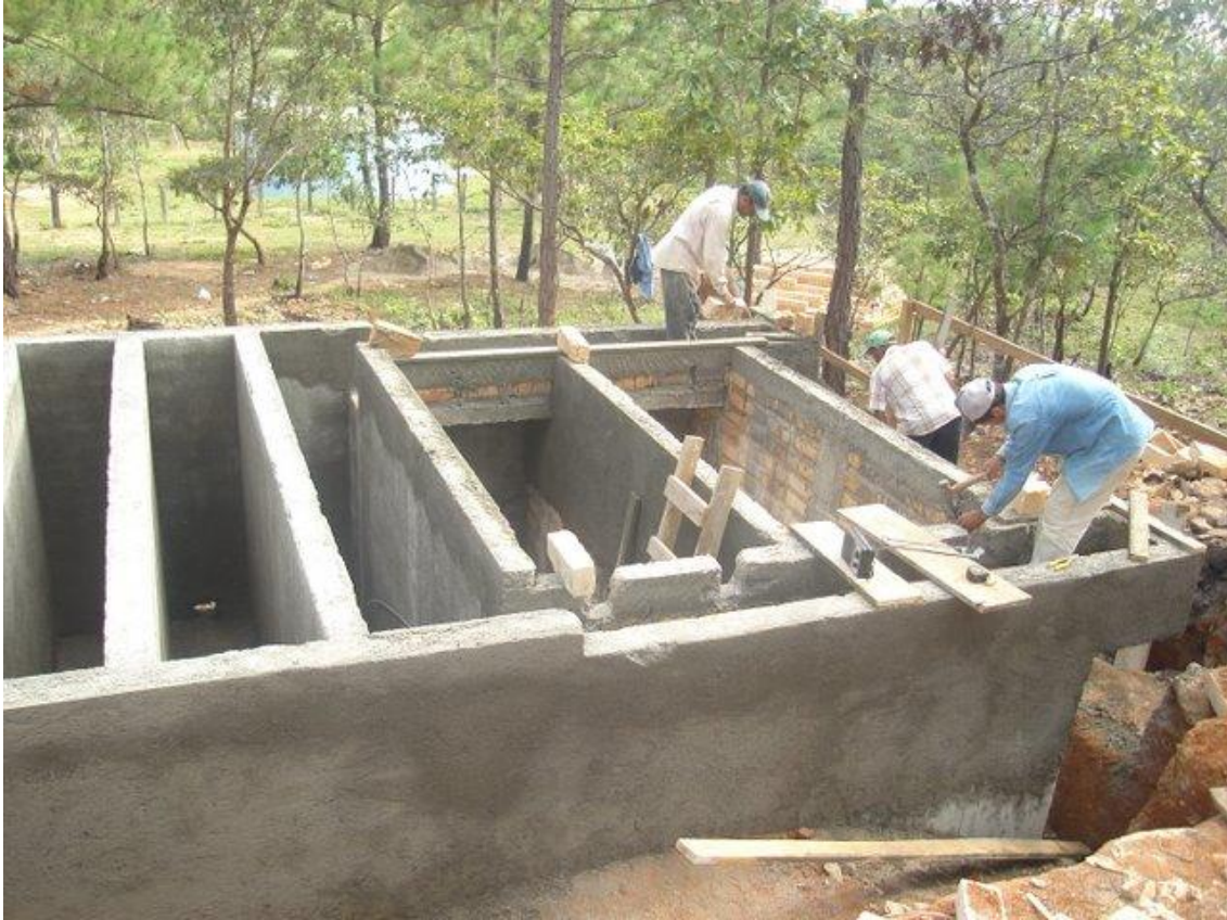
Construction of AguaClara water treatment plant
