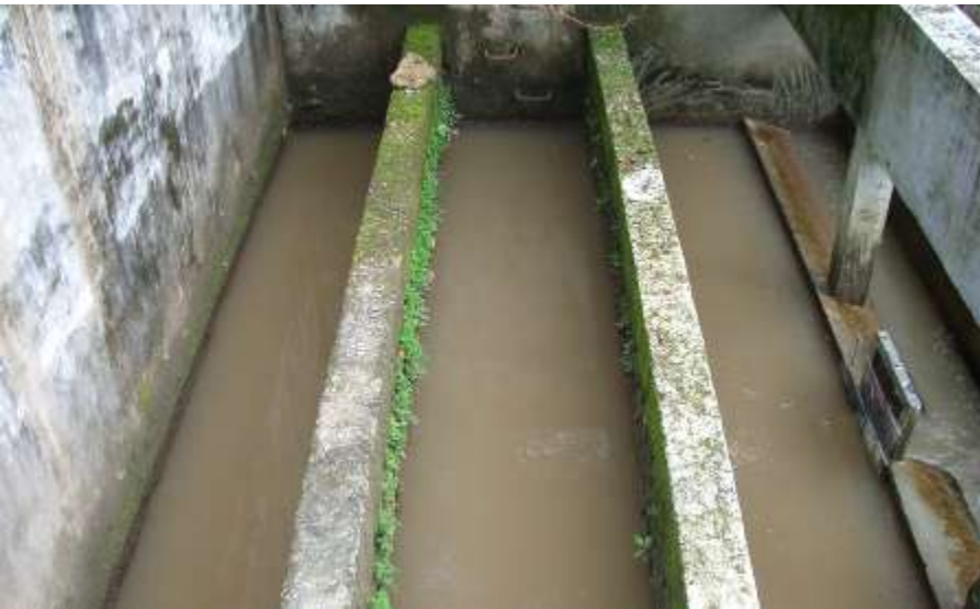
River water that is about to be chlorinated (Tela, Honduras – January 07)
