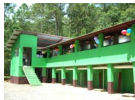
AguaClara water treatment plant in Marcala Honduras designed by CEE students.
