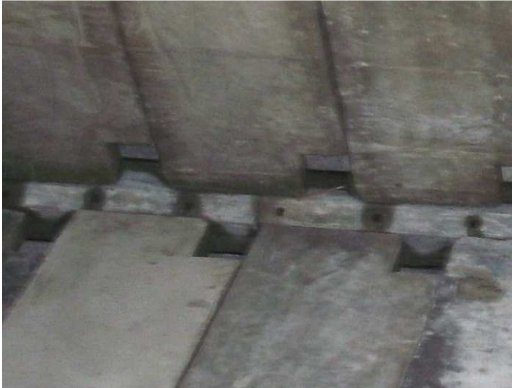
Figure 11: Staggered orifice and ports
