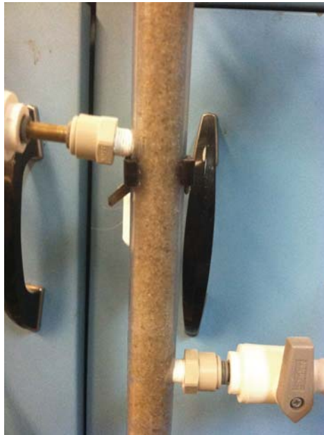
Figure 6: SRSF after soapy water test
